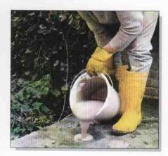
after mixing. If prepared with the correct quantity of water the slurry can be easily poured into the drill holes.
