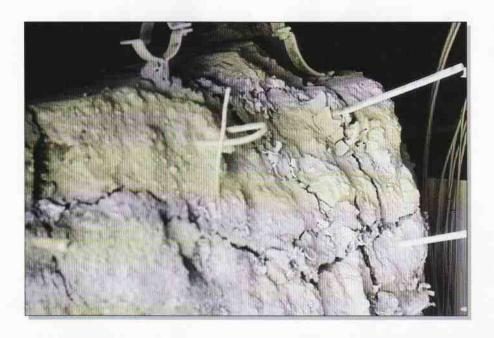
KATROCK is a non explosive demolition agent for use where explosives or mechanical means are not safe or practical. It can be used at concrete, rock or dimension stone.
